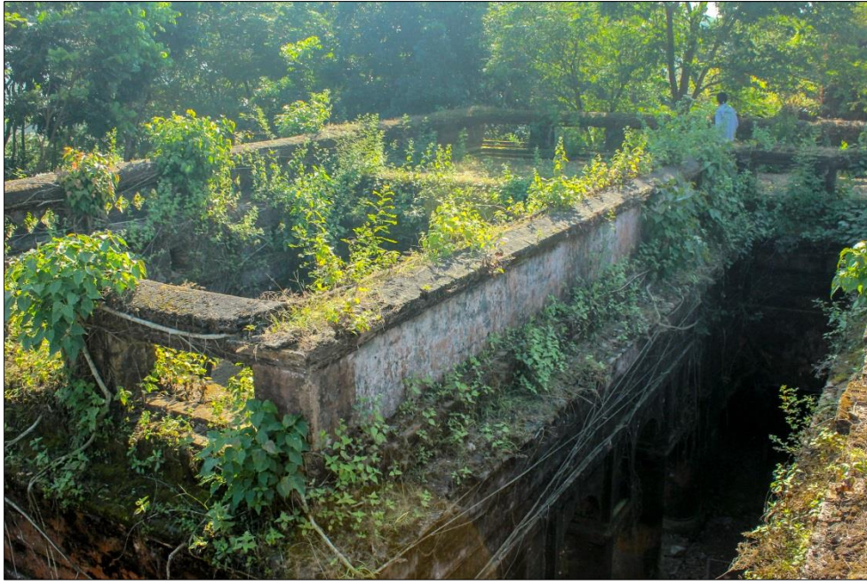
Pic: Roof Area
